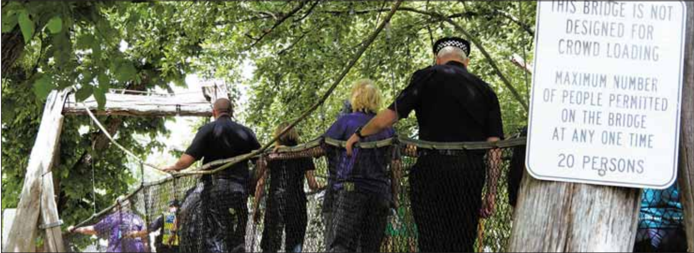
Walkers crossing the swing bridge over UT Creek. -AR
