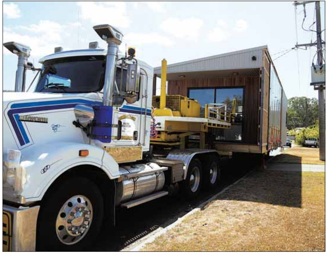
One of the homes about to be put in place. -AR
