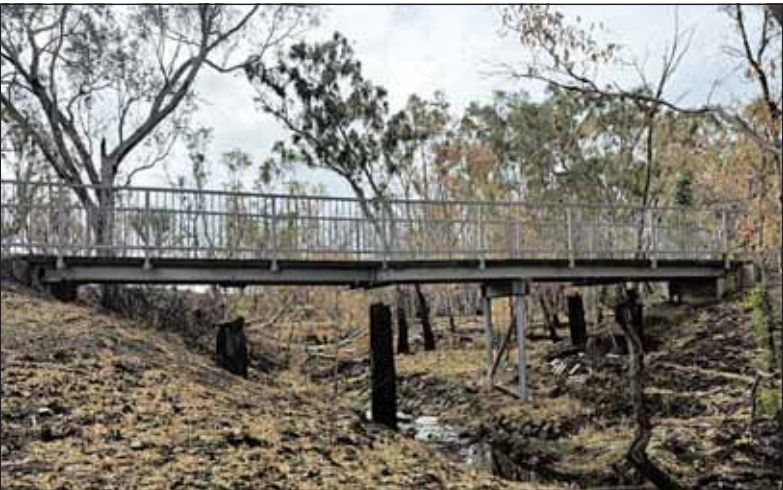
The underside of the bridge at Kanumbra. -S
