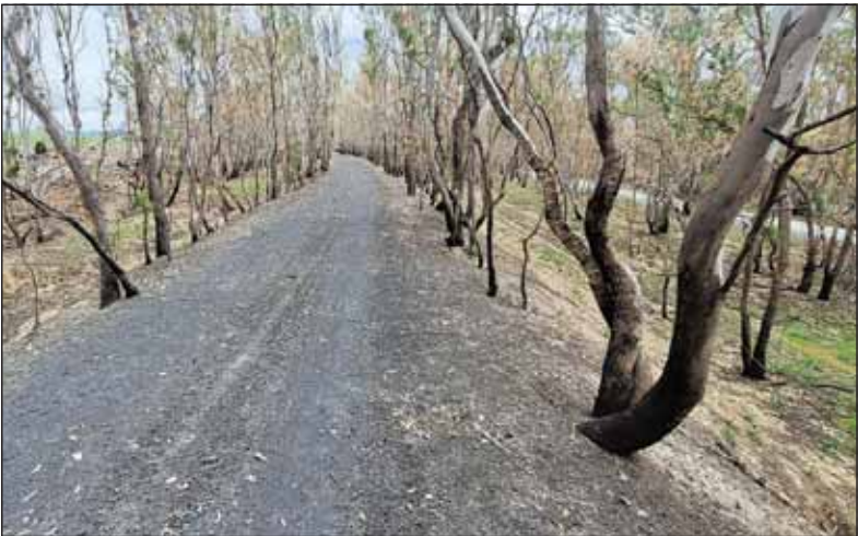
A surface view of the culvert. -S
