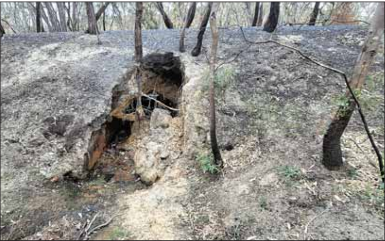
The underside of the culvert. -S
