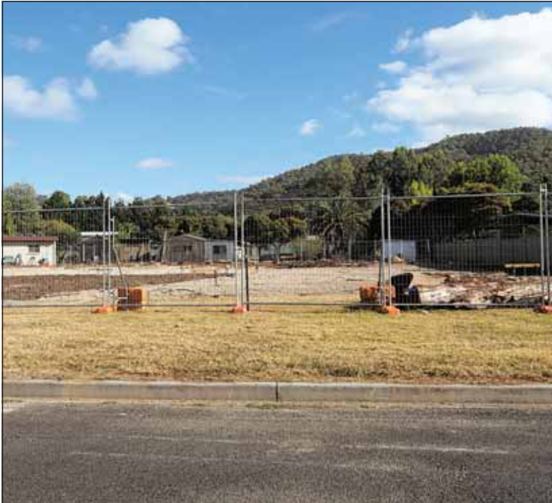
The Twenty-First Street site early on February 18, prepared for the arrival of the houses. -S
