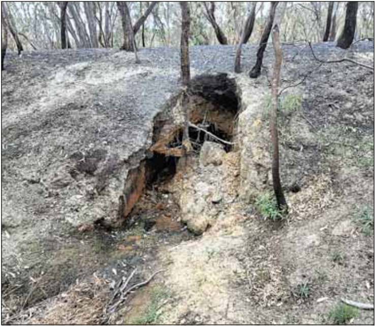
The underside of the culvert. -S
