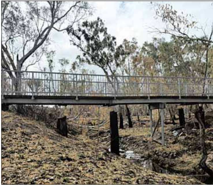
The underside of the bridge at Kanumbra. -S
